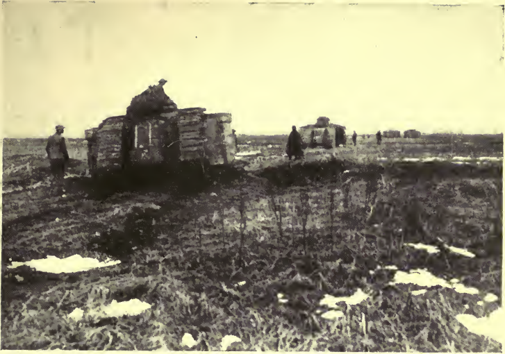
TANKS IN ACTION
