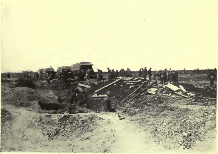
VICTORY'S HIGHWAY: LAYING THE ROAD OF PURSUIT OVER VIMY RIDGE
